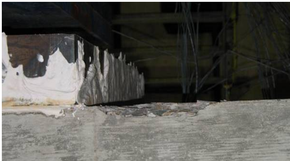
Figure 4-11: Photograph of compression block crushing
