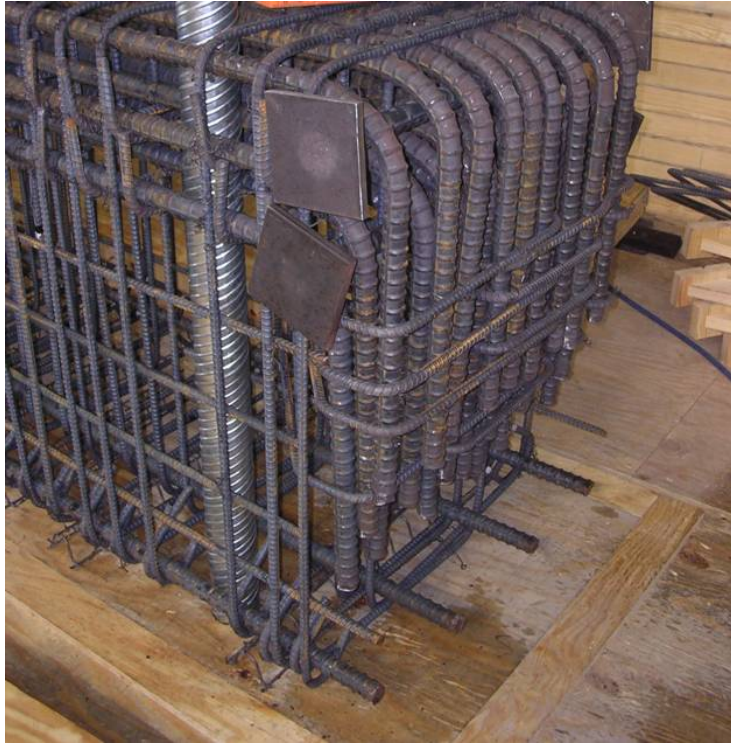
Figure B-3: Anchorage detail photo
