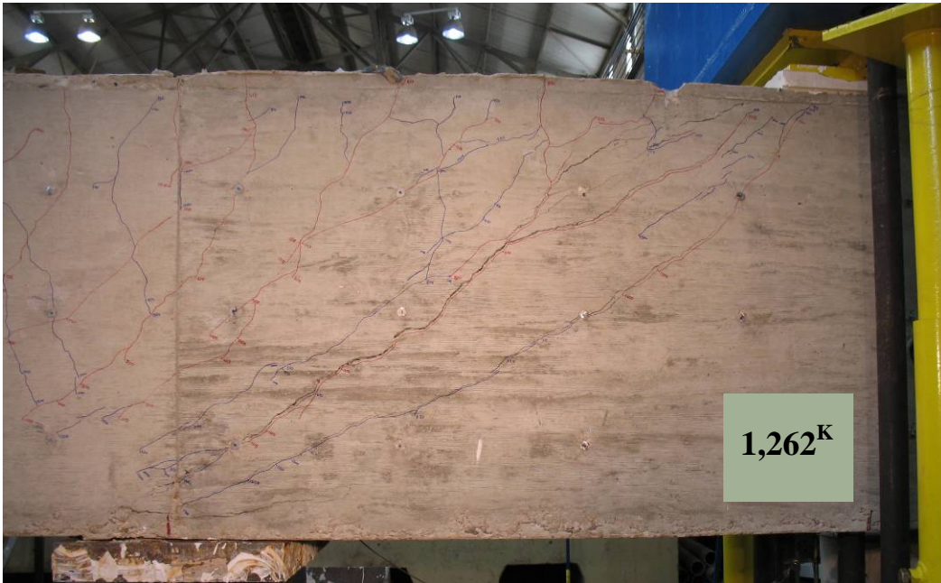
Figure C-5: Test #9 shear failure
